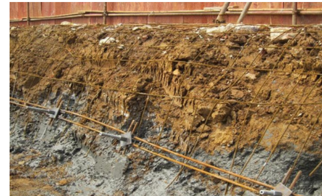
Nanjing Zijin investment side slope support
