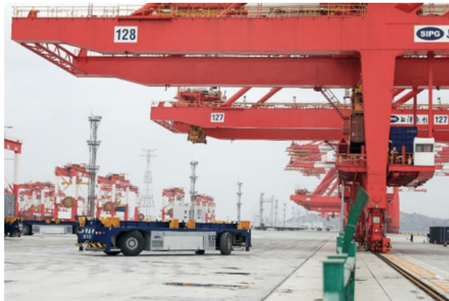
Shanghai Yangshan Port Automation Wharf Project
