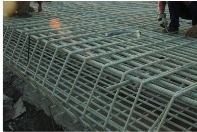
Cross-river tunnel underground continuous wall project
