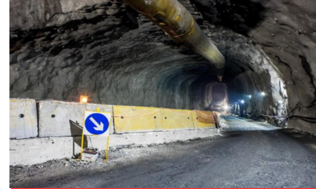
Jurong Island Tunnel in Singapore
