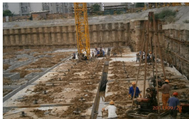
Army Command College anti-floating anchor
