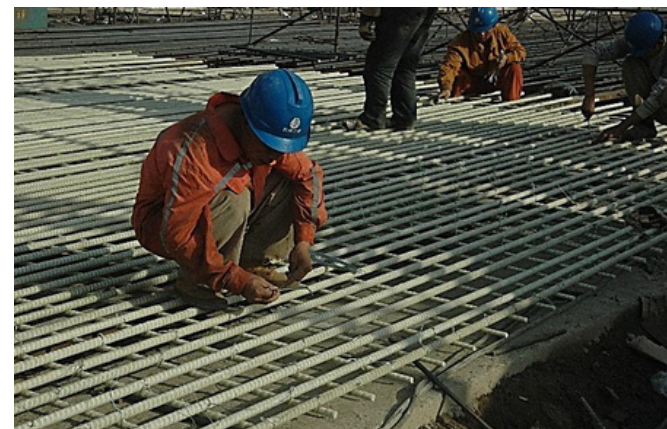
Subway Connecting Wall Project
